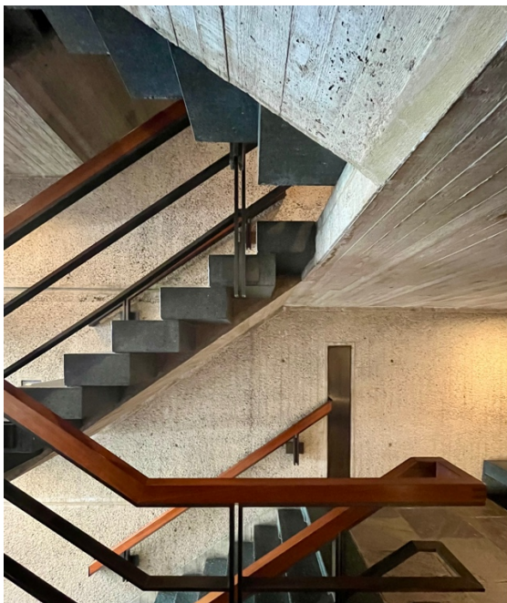
Staircase View looking north Photo: John Arbuckle August, 2023
