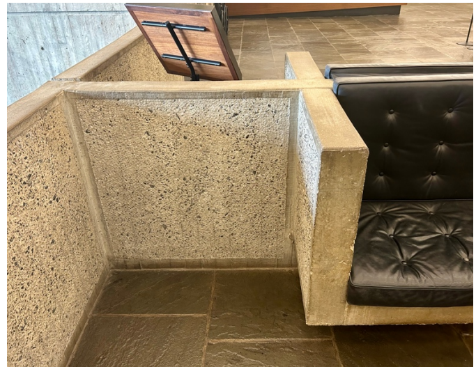
Lobby Bench detail Photo: Sean Khorsandi August, 2023
