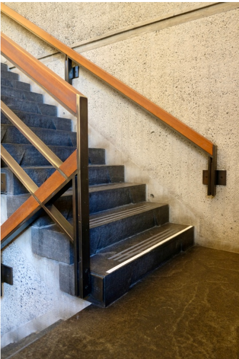
Lower Level View of stair looking southeast Photo: John Arbuckle August, 2023
