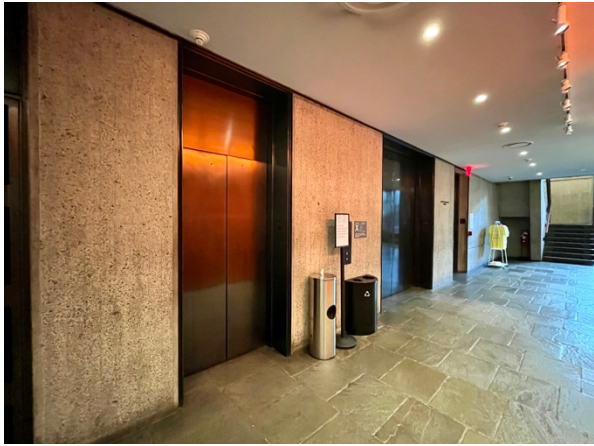
Lower Level View of Elevator Doors looking southwest Photo: John Arbuckle August, 2023
