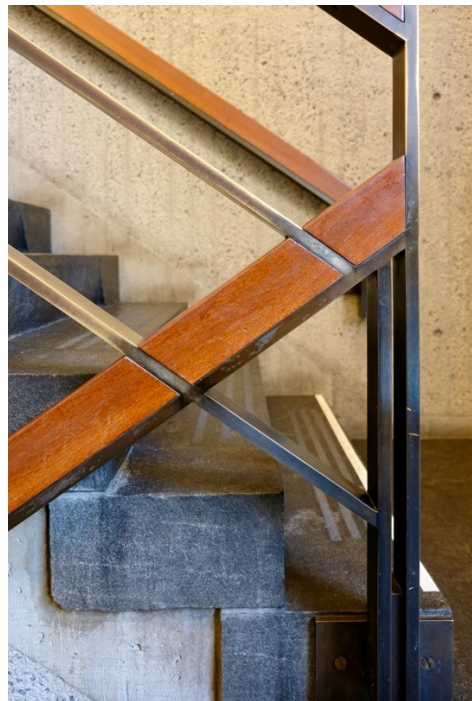
Lower Level Stair detail Photo: John Arbuckle August, 2023
