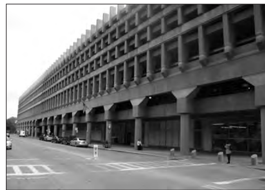
“Motorgate,” the parking garage at the terminus of the bridge connecting the island with Queens, Kallman & McKinnell, 1974.
