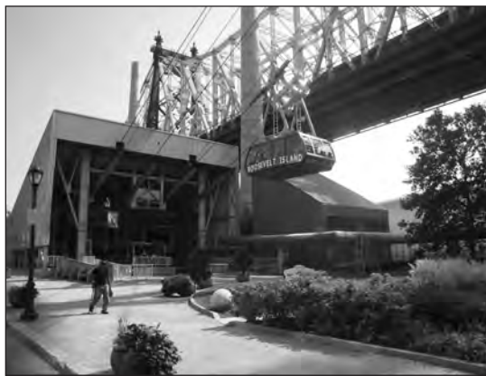
Island-side tram station, Prentice & Chan, Ohlhausen, 1976. The entire tram system was recently renovated.
